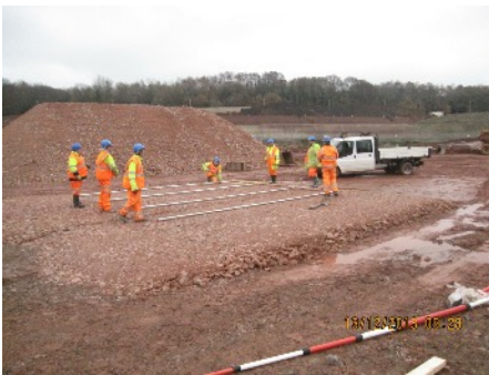
A trial assembly of the culvert units took place to ensure each member of the team understood the process as these were time critical works.
