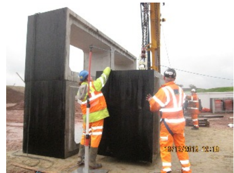
A trial assembly of the culvert units took place to ensure each member of the team understood the process as these were time critical works.
