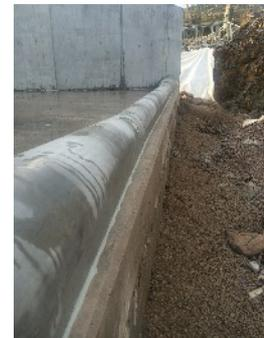
These photos show the toe beam being installed, the insitu reinforced concrete slab being poured and the external baffles on the inlet slab being installed.
