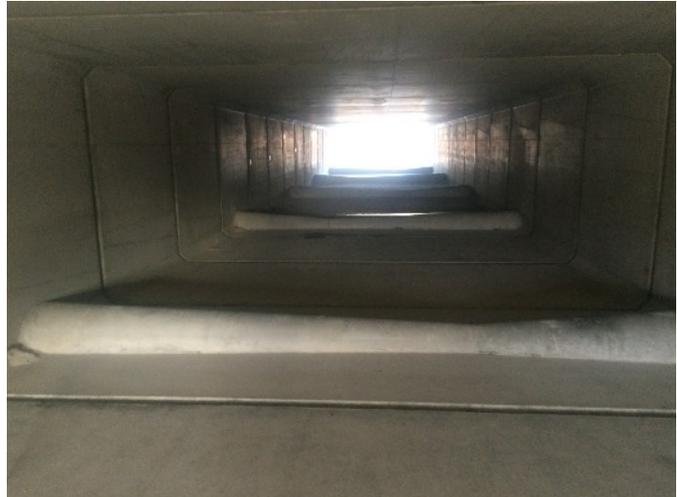
The photo above shows the inside of the culvert units after the external waterproofing was completed. Once the inside of the culverts was completely dry, the internal joint sealing could begin.
