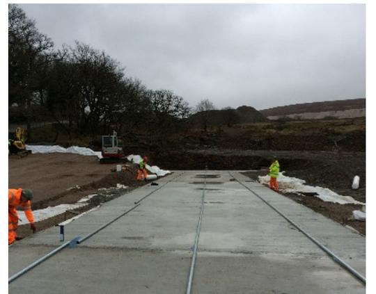
The photos below show the start of the culvert installation process. MDA used a 200T mobile crane to lift the units into place. The PCC units were delivered by Shay Murtagh on a 'Just in Time' system and were unloaded from the wagon and lifted straight into position. The wing walls were sat upon a PCC toe beam that acted as a lateral restraint for the culvert structure. These toe beams had starter bars that tied into the insitu RC inlet and outlet slabs which can be seen on the following page.
