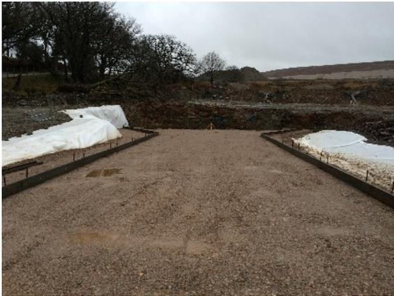
These photos show the preparation of the works area including installing the sub-base layers, mass concrete blinding, and the installation of the 6L sand layer prior to the culverts being installed.
