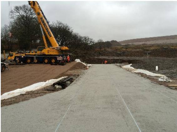
It can be seen from the photos below that MDA use a system of installing aluminium tubes within the sand layer which assists when positioning the large 27 tonne culvert units.
